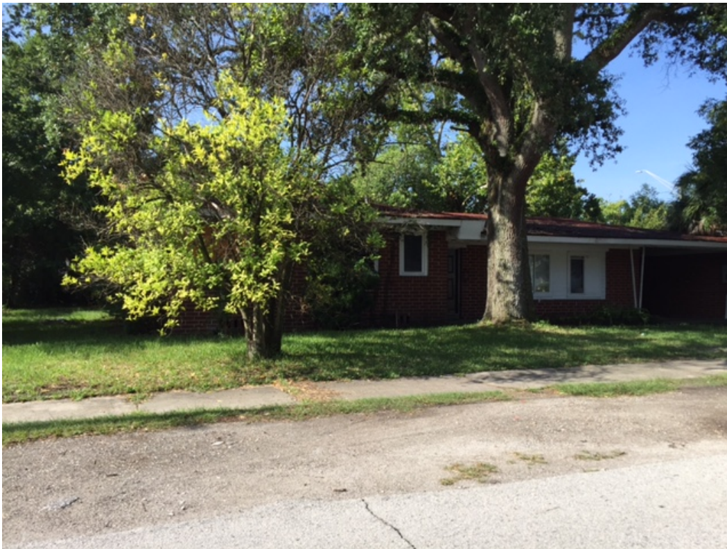
View of site with vacant dwelling.
